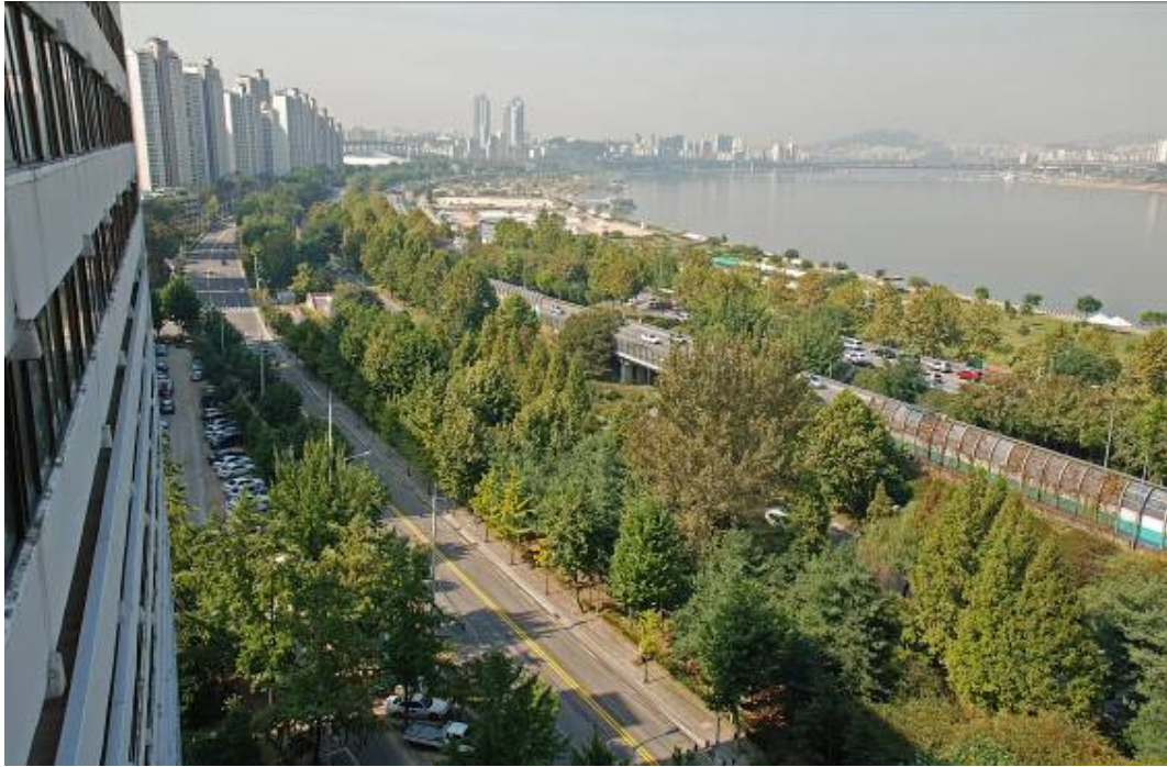
Fig.5 The healthy growth of trees, like Metasequoia , Populus , etc. betrays the abundance of fresh, subsoil water, under the parapet-walls of the apartment blocks along the river Han.
